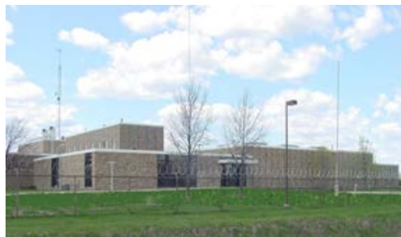
City of Oregon Water Treatment Plant
